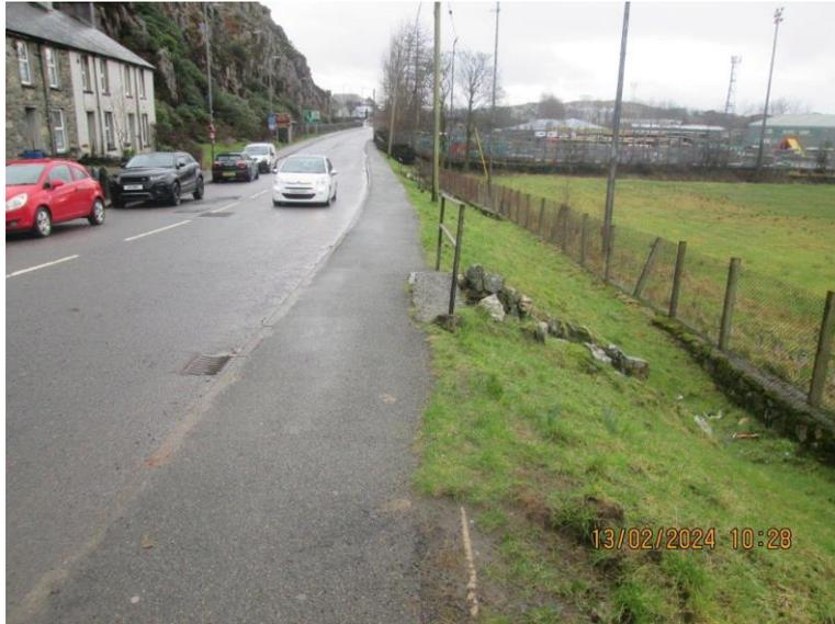
**Photo 5:** A470(T) Llwyn y Gell Road Southbound adjacent to Bro Ffestiniog Rugby Playing Field. – proposed cycle track widening in existing grassed embankment location
